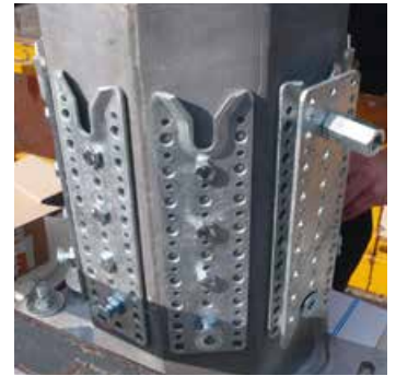
Ridge node for dome roof
