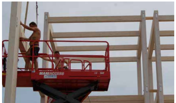
Installation of the secondary beam using RICON® S.
