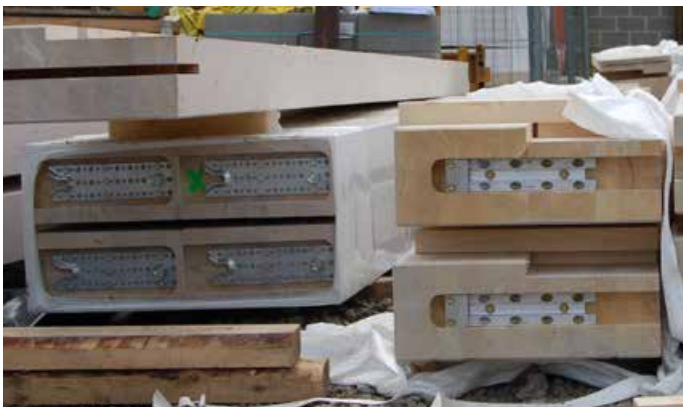
RICON® S installed in end grain, concealed on three sides.
