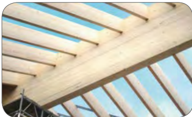
Hall roof of carpentry S. Hinrichsen (Germany)
