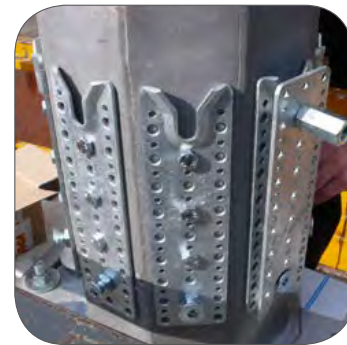
First node for dome
