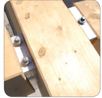
Connection finished: The secondary beams are placed in the clamping jaws.
