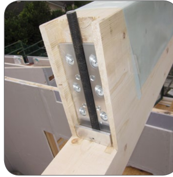
Concealed mounting on three sides by milling the secondary beam and visible mounting on main beam.
