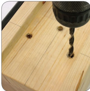
2) Pre-drill screws (see installation instructions).
