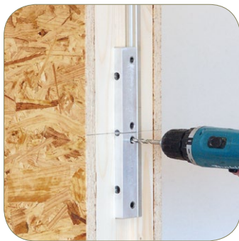
1) Predrilling with drilling-jig
