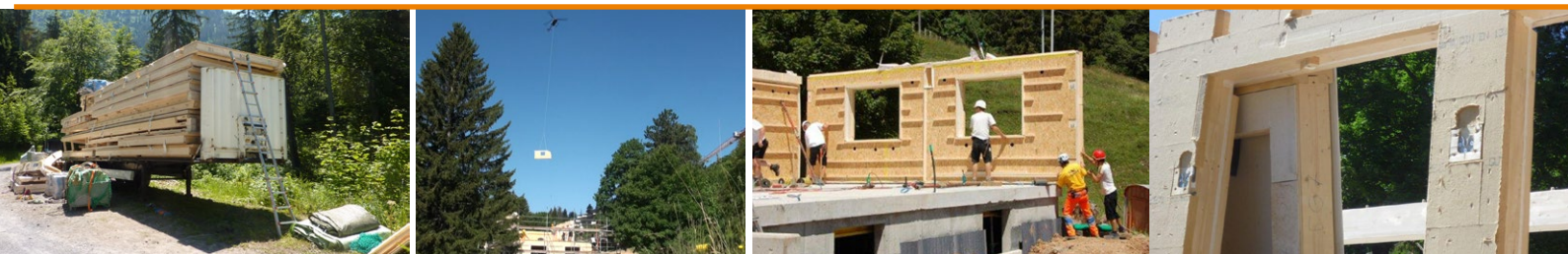
Helicopter assembly | House on the Rigi (CH)
