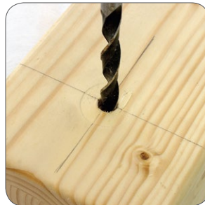
2) Pre-drill screws (see installation instructions).
