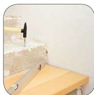
2) Gluing and install
