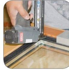
3) Screwing or nailing the FIXclip-Profile
