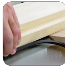
4) Press in wedge-shaped sealing
