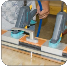
2) Pressing pane of glass against outer seal
