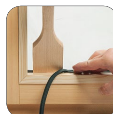
4) press in the wedge seal
