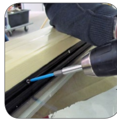
2) Fix FIXclip-Profile with nail/screw
