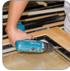
3) Screwing or nailing the FIXclip-Profile
