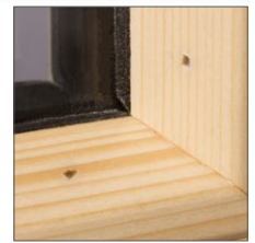
Usually, glass bar is attached with exposed nails.
