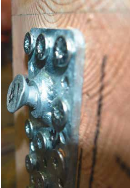
Figure 13: Collar bolt yielding in beam member
