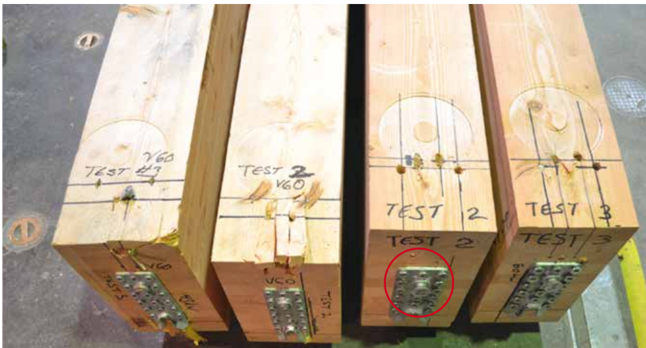
Figure 10: Example of collar bolt yielding at maximum drift and load in beam member RICON® S VS 200x80 in 3 out of three tests
