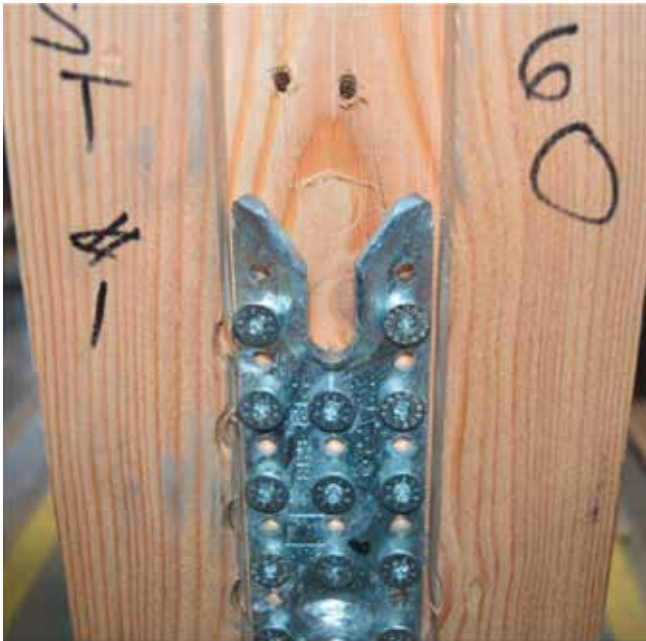
Figure 17: V-notch without damage on RICON® S VS 200x60
