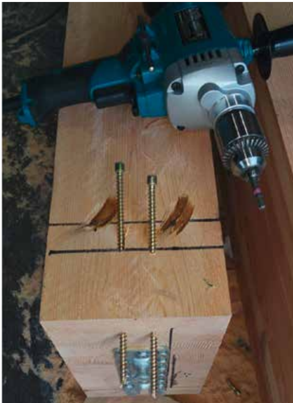
Figure 12: Example of uplift toe screw install
