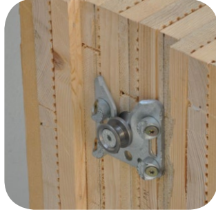
Connector plate with screwed double collar bolts
